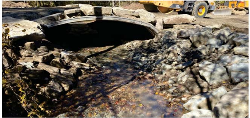
Stream Crossing Replacement in the City of St. Marys
