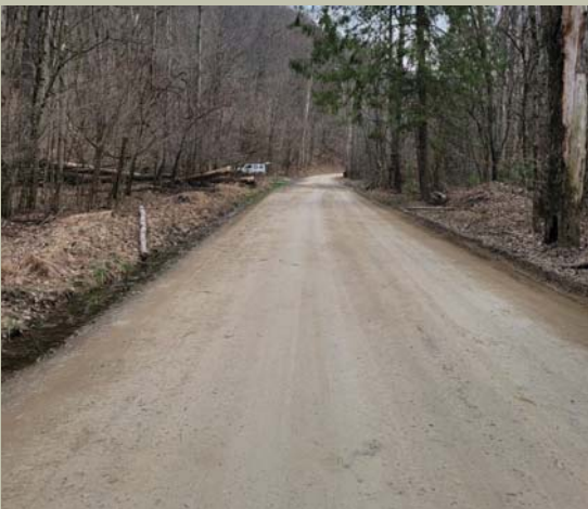
Medix Run Road before project
