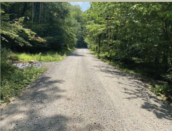
Medix Run Road after project
