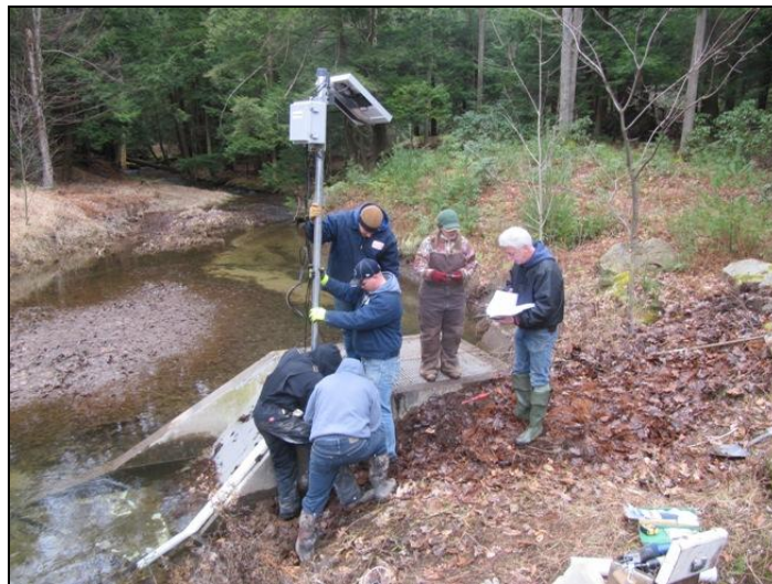
Satellite Telemetry Water Monitoring System Being Installed
