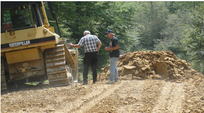
Stony Hill Road, Placement of Fill Materials
