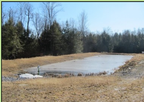
Pond that is lined with both limestone and a mushroom compost substrate.
