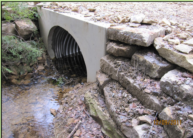
New Stream Crossing Culvert and Headwall
