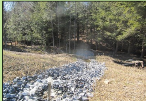
Treated water is directed back into the stream channel via a limestone rock channel.
